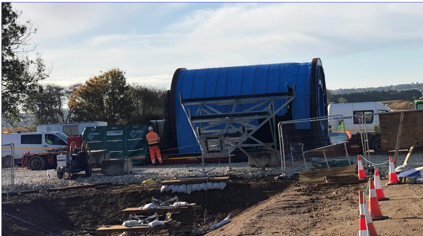
Figure 4.5: Cable Drum Delivered to Site
